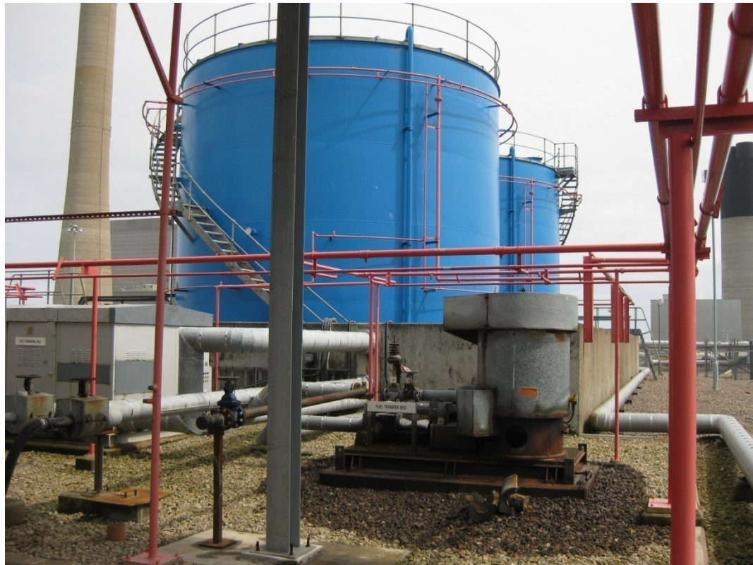
Photo 3.7: No. 2 Distillate Fuel Tanks and Forwarding System
