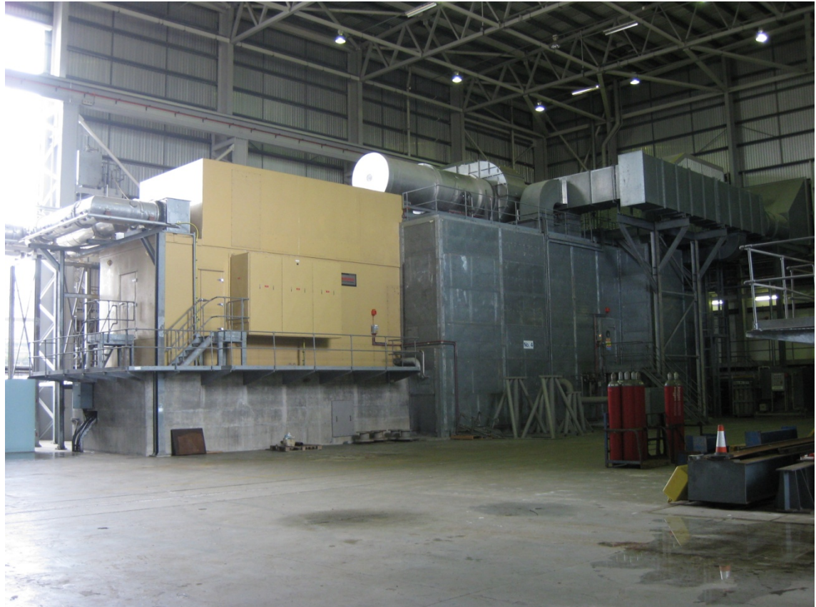
Photo 3.3: Frame 9 Unit Inside Building
