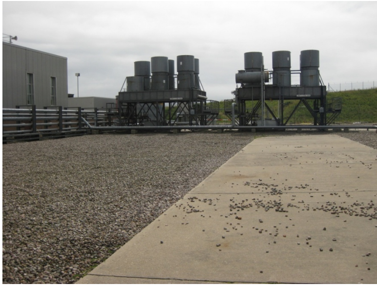
Photo 3.8: Fin Fan Cooling Skids (One Per Unit)
