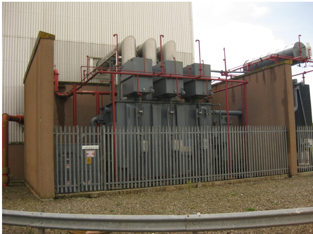
Photo 3.10: Main Generator Step Up (GSU) Transformer
