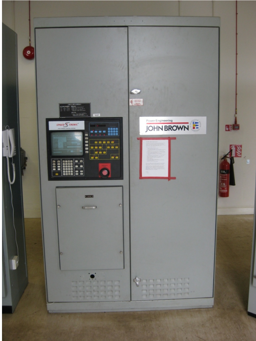
Photo 3.4: Speedtronic Mark IV Panel
