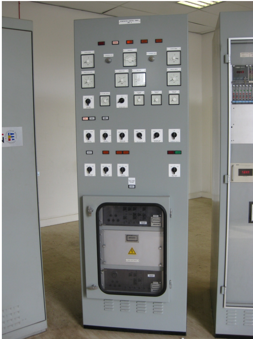
Photo 3.5: Generator Control Panel with MAVR.
